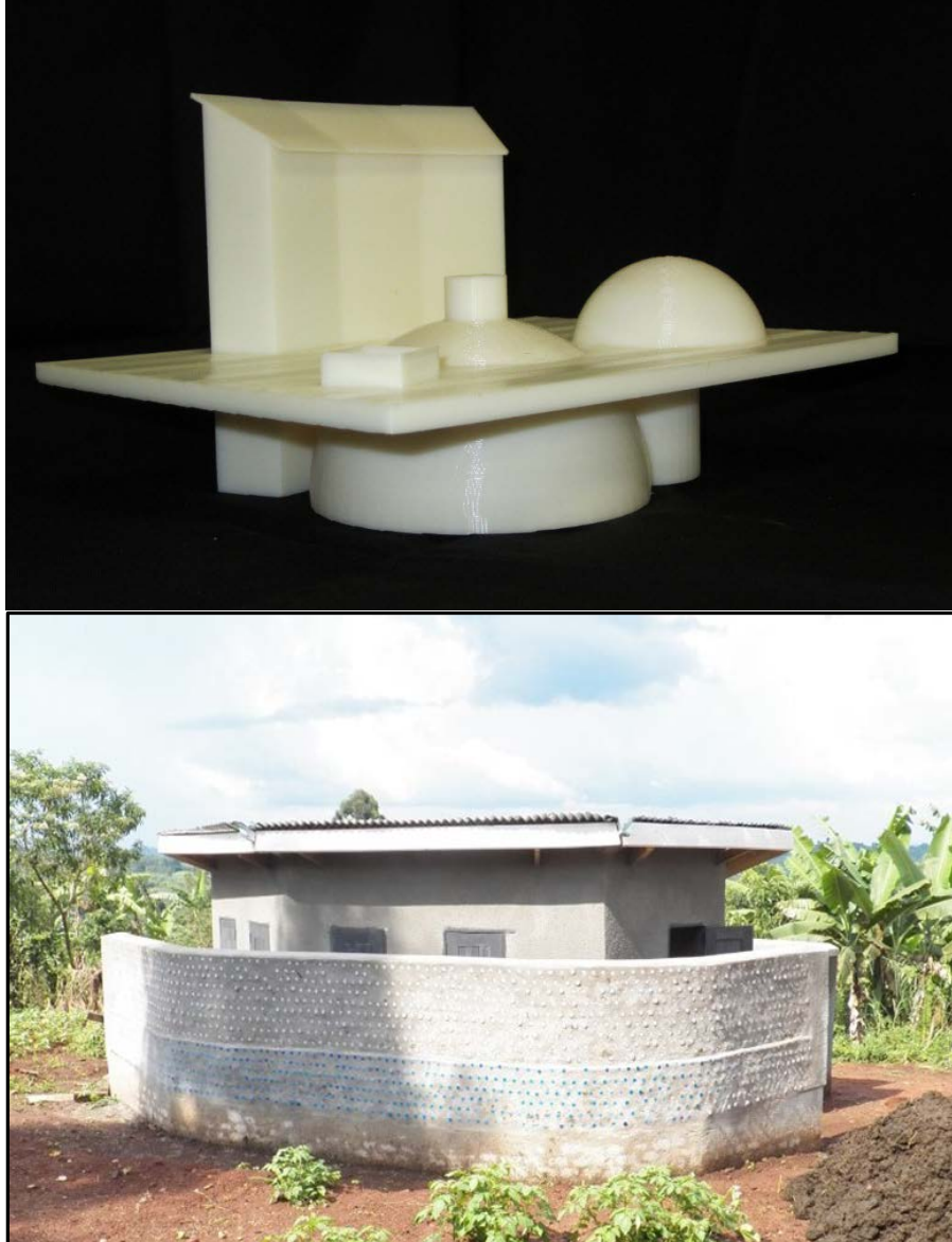
Figure 7: Latrine-based Biogas System. This design (top) was created to communicate the components and concept of a biogas digester build at a rural school in western Uganda. The horizontal plane (x-y plane) shows the relevant perspective of the ground surface to delineate the aboveground and subsurface components of the system. The final constructed latrine (bottom) is operational and produces biogas used to fuel the cook stove in the school kitchen. The combination of 2D images and 3D models has been used several times to describe this outreach project completed as part of a student research project.
