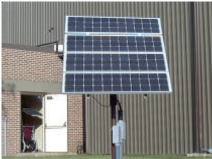
Figure 2. Solar Array assembly.
