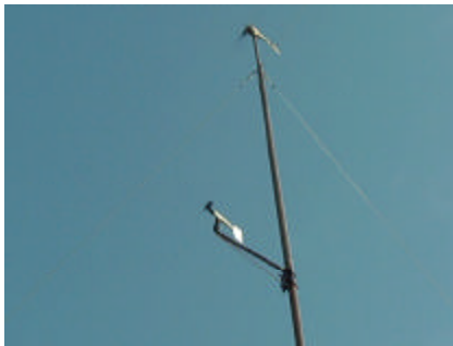
Figure 3. Mast mounted wind generator.
