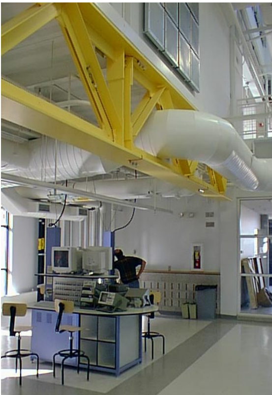
Fig. 3 40-foot truss has vibrating wire strain gauges at 10 locations
