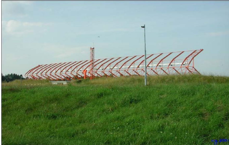
Figure 6. Typical localizer antenna installed at runway end.
