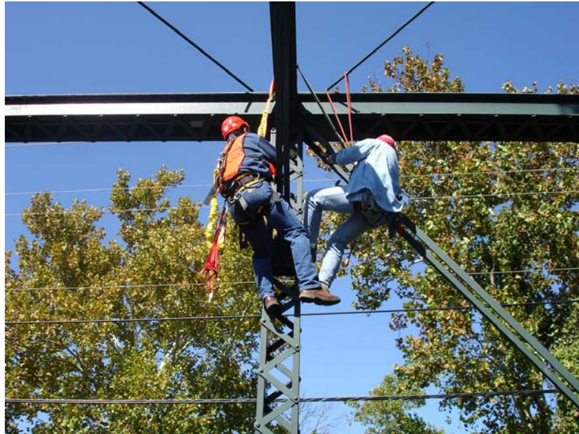
Figure 5. Inspection of a Joint Connection
