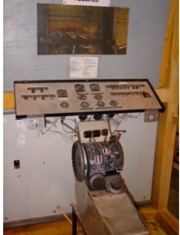
Figure 6 Control Panel for Texas State Technical College
