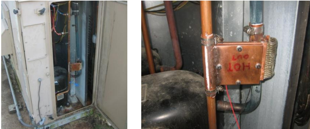
Figure 6. The photographs of the TEG module clamped to the pipes of the compressor
