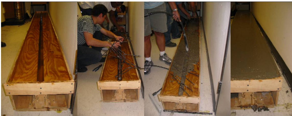
Figure 8 Construction of the Reinforced Concrete T-Beam
