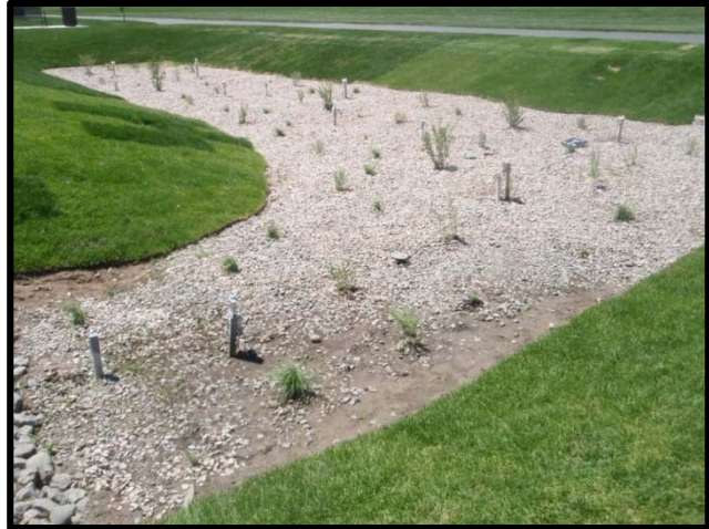
Figure 2. Rain garden in Cottonwood Heights, Utah as an example of green infrastructure elements that require interdisciplinary knowledge and skills bridging geoscience and engineering.
