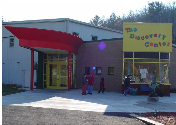
Figure 1. Discovery Center (Front Entrance)
