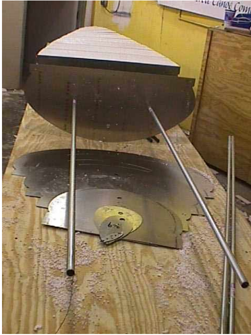
Figure A1. CAD/CAM designed and machined frames for the Concrete Canoe mold.
