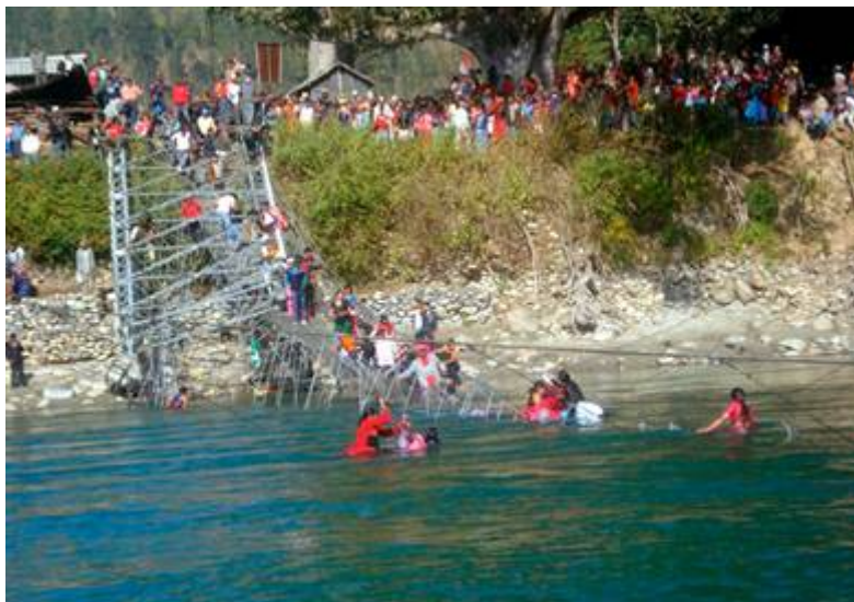
Figure 2—Failed bridge in Nepal that had been built by a non-profit agency 13
