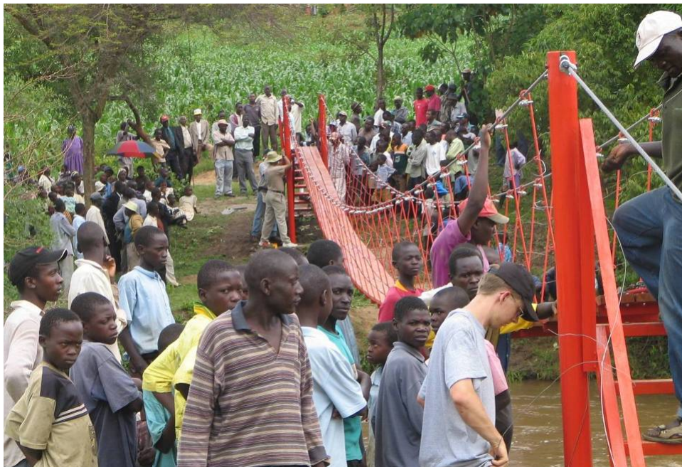
Figure 3—Building a bridge over the Sand River in Western Kenya 12
