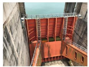
Fig. 9. The overflow gate of the Hòa Bình hydropower plant.
