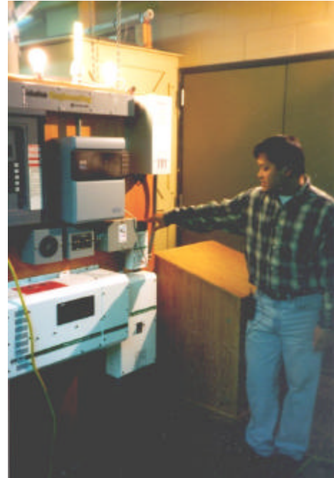
Figure 4. Cesar Salire with inverter and control panel
