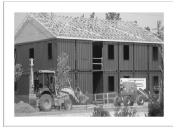
Fig. 15: Use of Shipping Container
