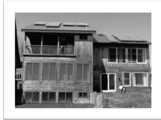
Fig. 20: Use of photovoltaic on the roof in Eco-village, New York 18
