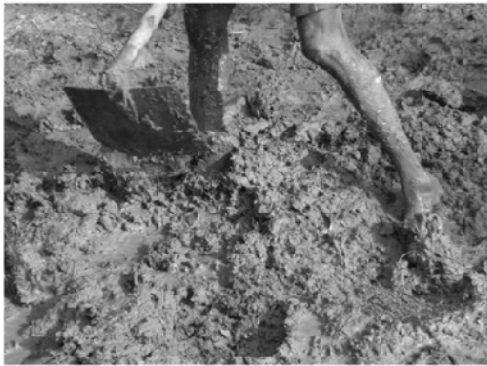
Fig. 8: Mixing of Mud 12
