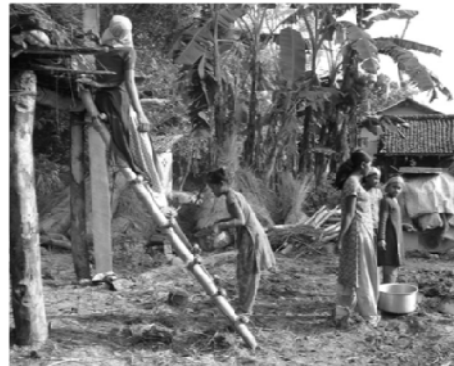
Fig. 9: Mixing a Mud 12
