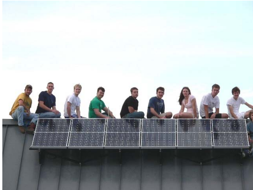
Figure 1. Students pose for a picture after installing six BP7185 185W (peak) PV modules and a powder-coated steel mounting structure on the Museum's standing-seam roof.
