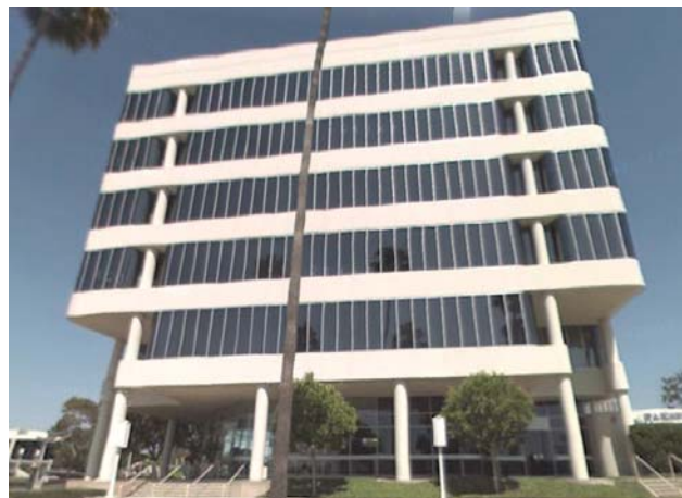
Figure 1: Overview of building geometry and architectural features of its facade
