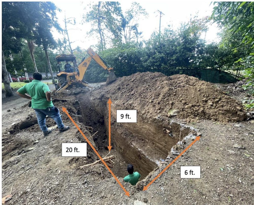
Figure 5: Initial Location of The Trench
