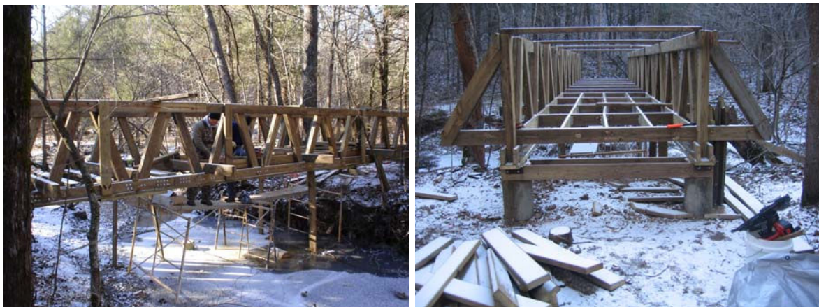
Figure 4. Partially completed bridge superstructure showing ongoing construction in freezing weather conditions.
