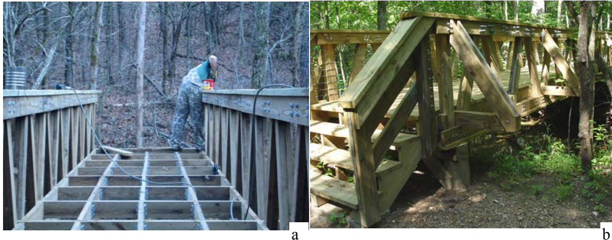
Figure 5 a). Completed superstructure. b.) Completed bridge.
