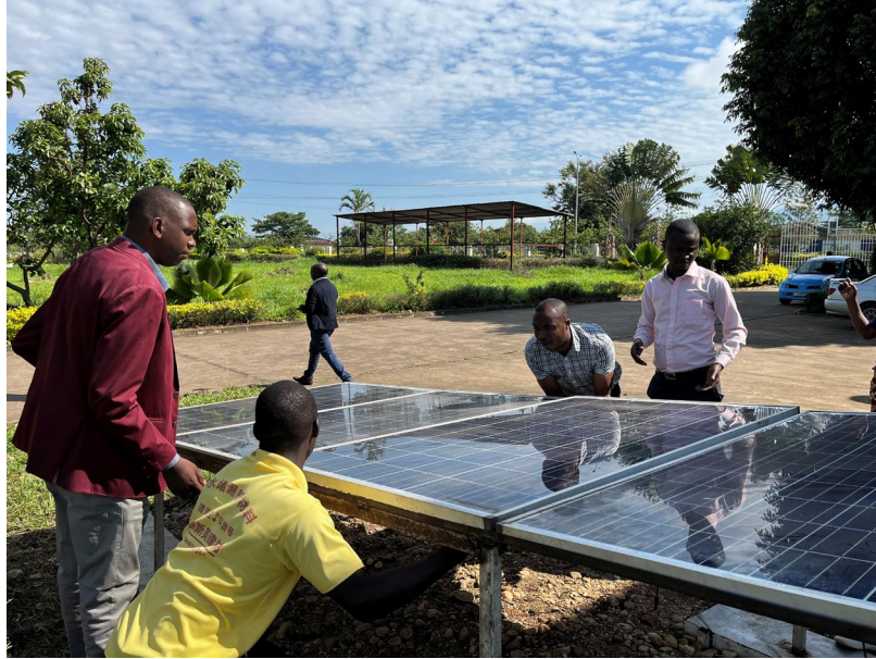
Figure 2. Professors and Electrician Wiring up Solar Panels
