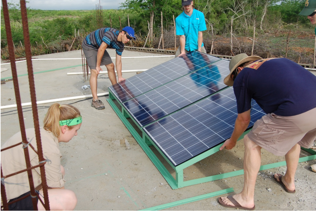
Figure 8 Working on the solar panel installation
