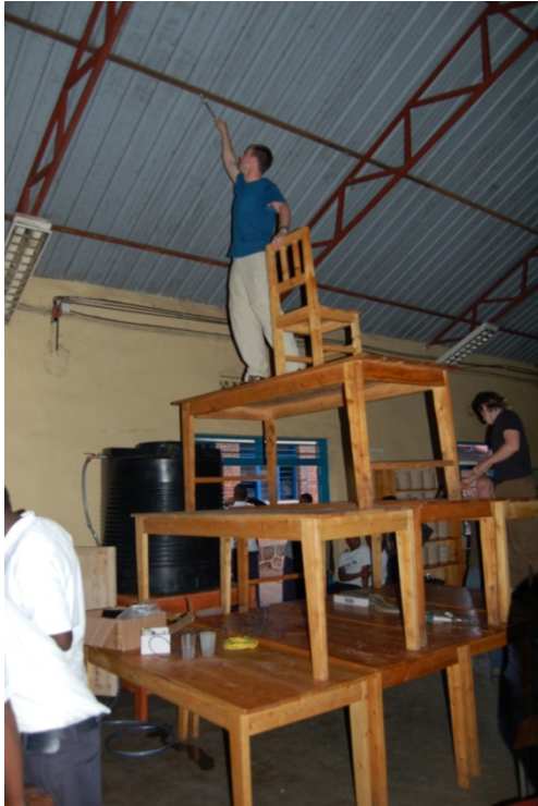
Figure 6 Installing the solar panels.
