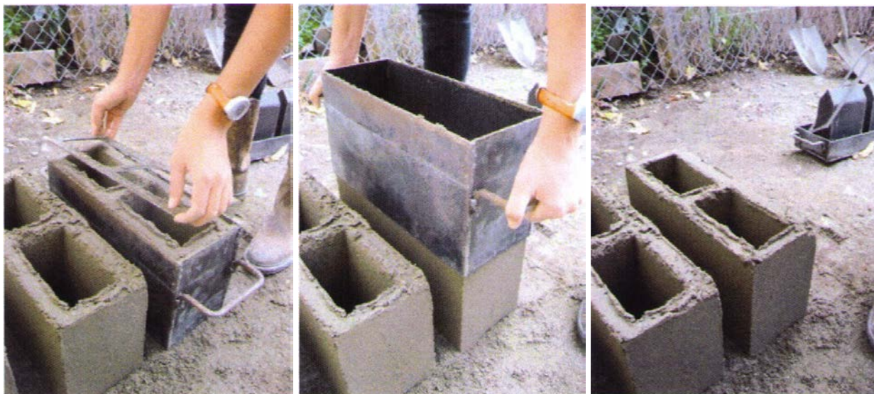
Figure 6: CMU Block Production (a) Removal of Base and Top Plates (b) Removal of Shell and (c) Final CMUs
