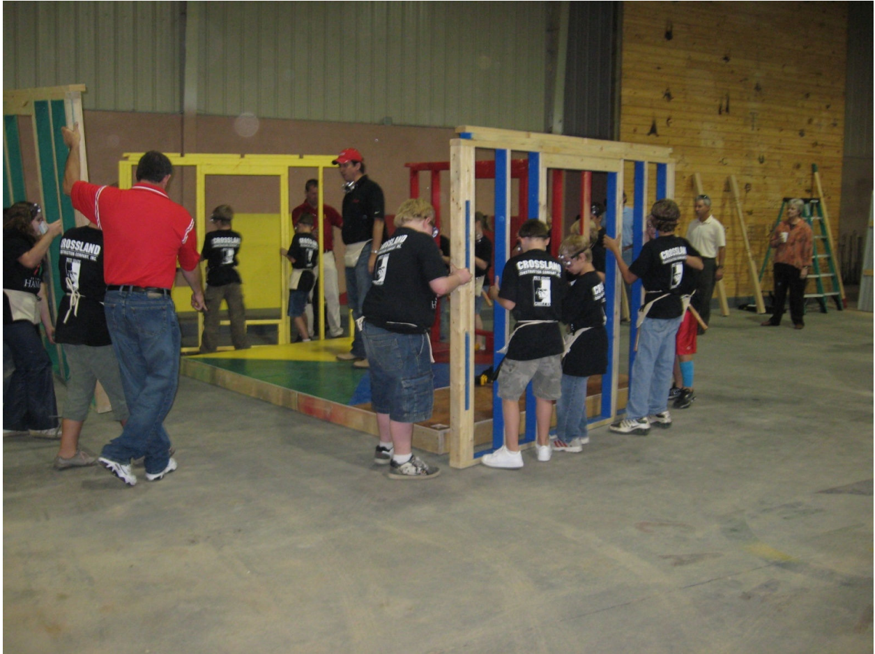
Installing wall framing
