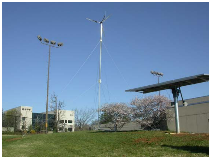
Fig. 6 Wind turbine and solar tracking PV array
