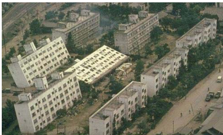
Figure 1: Tilting and settling of apartment complex in Niigata, Japan due to 1964 Niigata earthquake ( http://www.ce.washington.edu )
