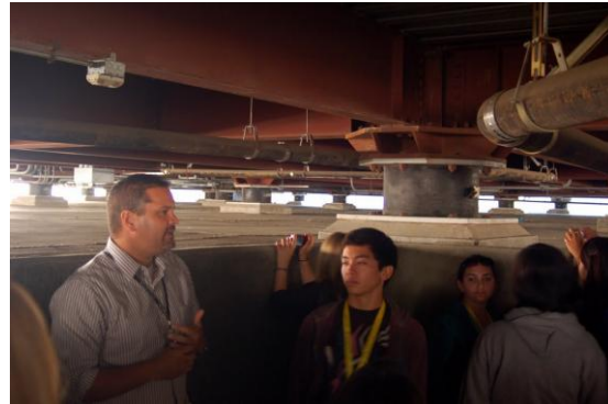
Figure 8: Base Isolation System at San Diego Office of Emergency Services building
