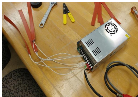
Figure 3. Heating pads connected to the power supply
