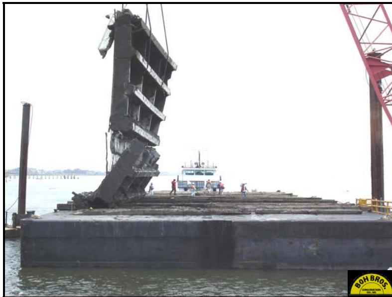
Figure 5: Submerged Deck Removal
