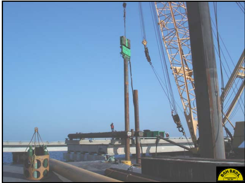
Figure 12: Pile Installation for Auxiliary Steel Bents
