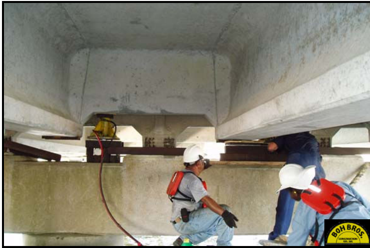
Figure 6: Vertical Jacking of Deck on to Teflon Slide Plates
