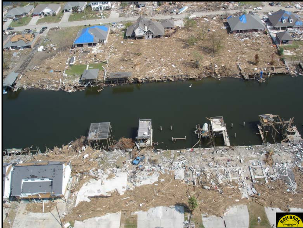
Figure 3: Infrastructure Damage – North Shore of Lake Pontchartrain
