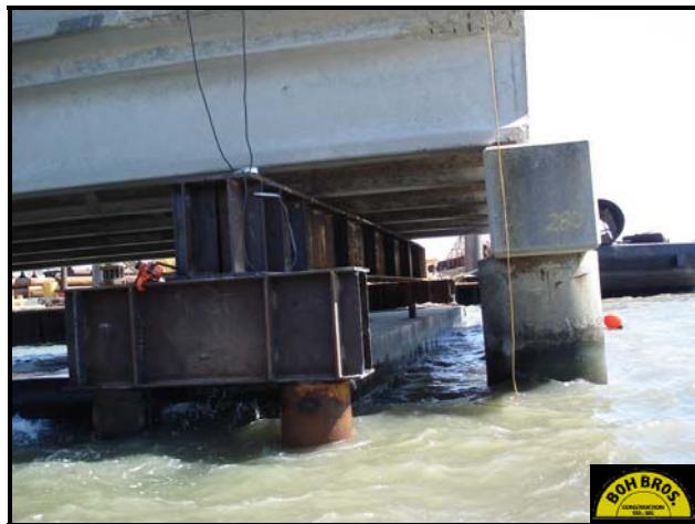
Figure 11: Auxiliary Steel Bent
