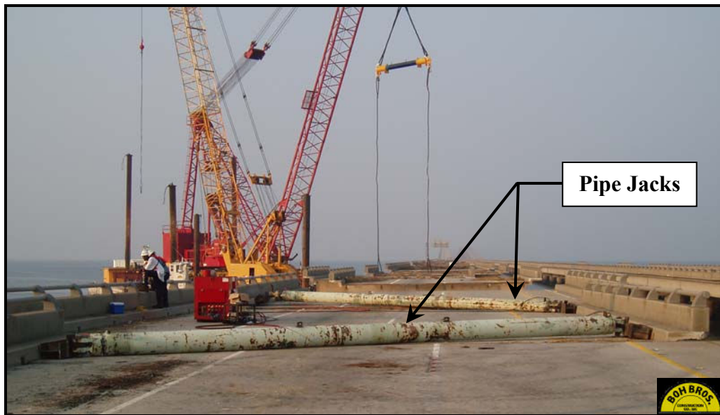
Figure 7: Horizontal Re-alignment Jacking
