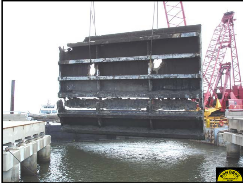
Figure 4: Submerged Deck Removal
