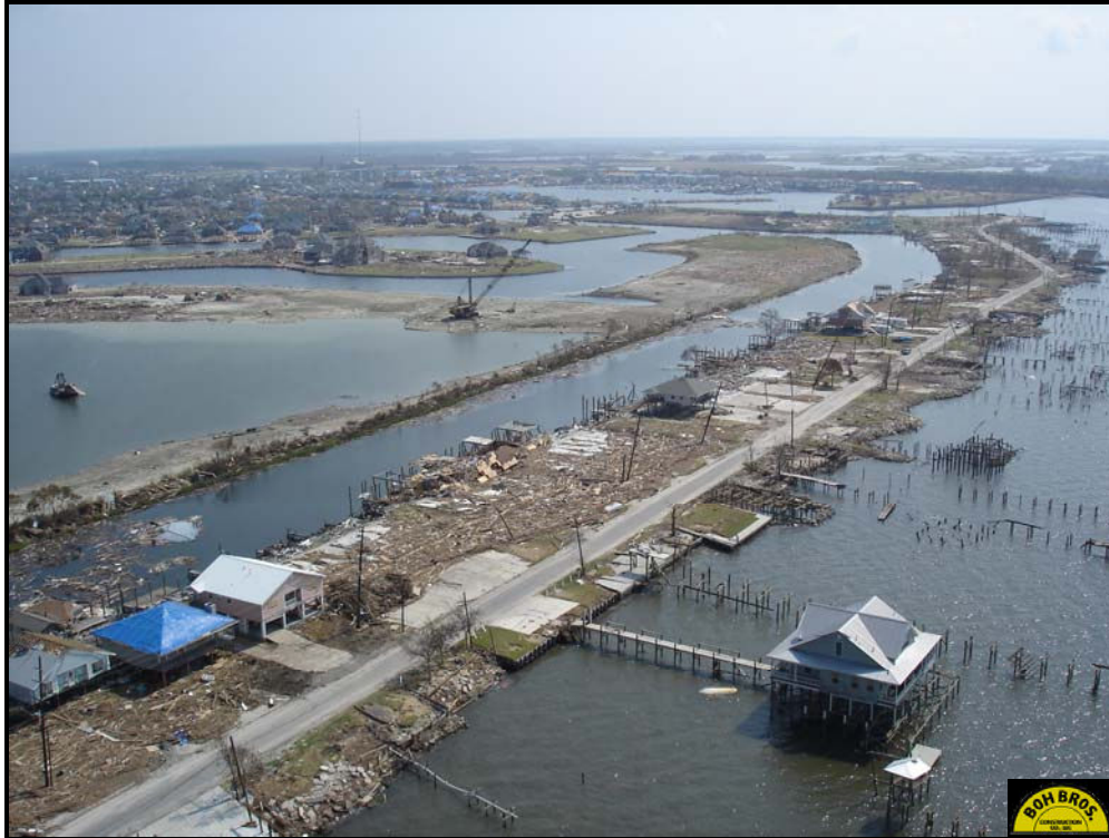
Figure 2: Infrastructure Damage – North Shore of Lake Pontchartrain
