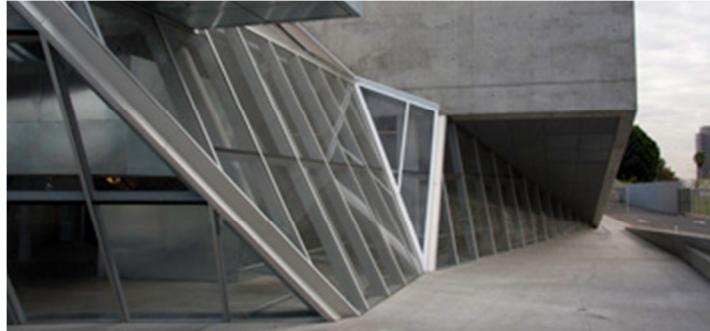
Figure 3: Stick-Built Glass Façade
