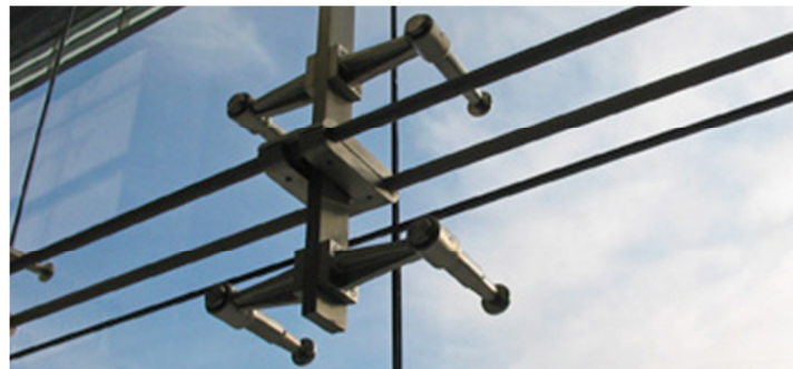
Figure 7: Bolted Glass Systems
