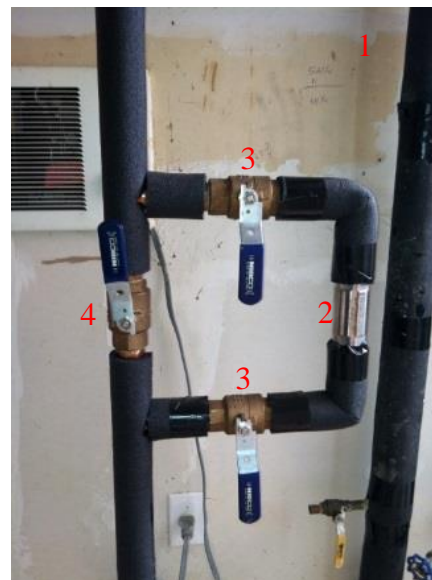
Figure 5a. Circuit Solver TRV and pay-pass valves
