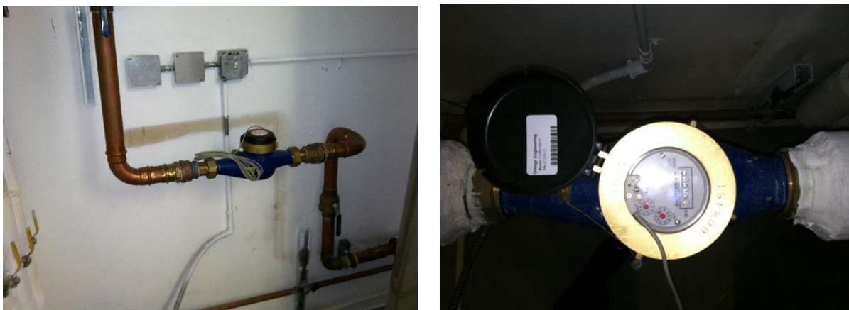
Figure 5d. New water meter to measure consumption with/without circuit solver TRVs [21]
