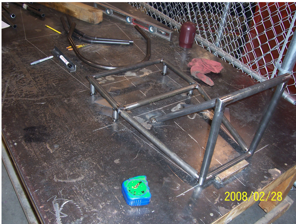
Figure 8: SAE Car Frame Weld Fitting
