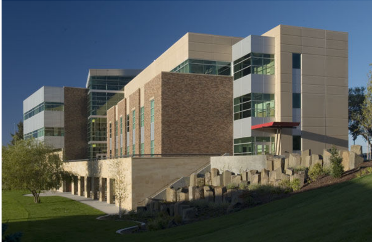
Figure 1, Computing and Engineering Building at EWU
