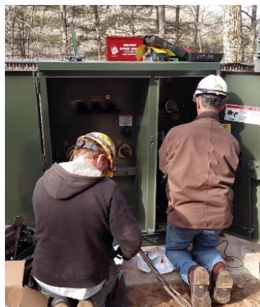
Figure 6: Wiring New Transformer
