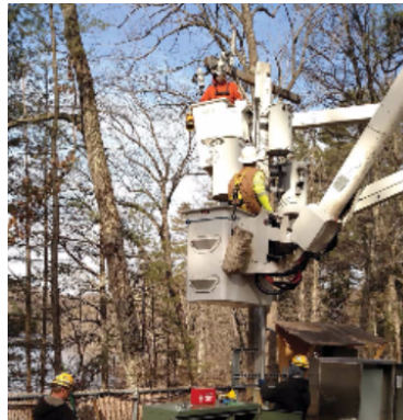
Figure 5: Old Transformer Removal
