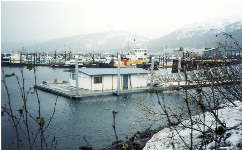
This 40-foot by 60-foot floating concrete fuel dock is located in Whittier, Alaska. The project involved wave forces, movement due to 30+ foot tide changes, buoyancy calculations, as well as concrete design, pile design, aluminum gangway design and the design of fuel lines, water lines, and power.
