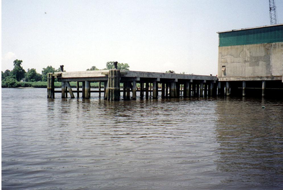
Photograph 2: Wharf Extension in Georgetown, South Carolina. This project required an evaluation of ship impact forces, seismic forces, heavy vertical loads from cargo and cargo transfer equipment, and protection of the materials from the corrosive effects of salt water.
