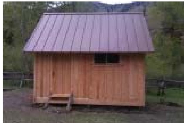
Figure 9. New power house.
