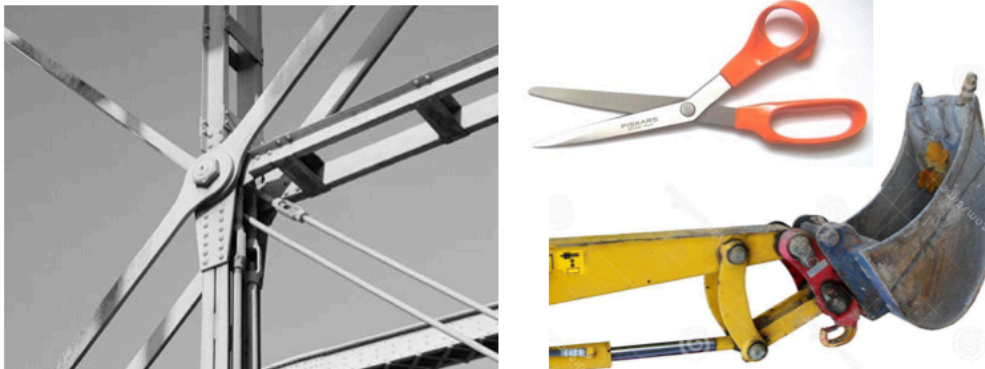
Figure 5: Common pin connections. Pins are often bolts or rods. These connections are useful when you want to allow for some rotation, but not all pin connections are designed to rotate. They are also relatively easy to construct.
