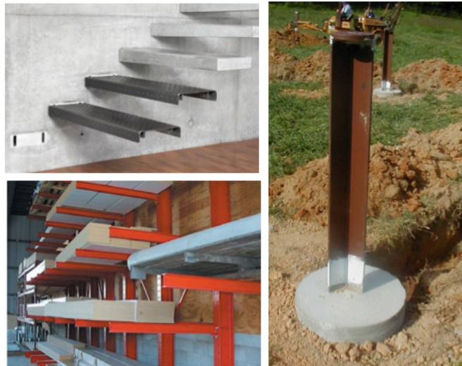
Figure 4: Fixed connections are key to any cantilevered member, whether it is a horizontal or vertical member.
