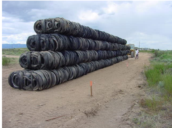
Figure 8: Prototypical Tire-Bale Wall for Noise Abatement
