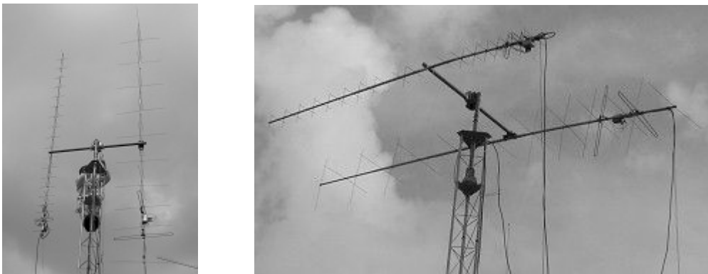
Figure 4. AMSAT antenna refurbishing, part of the ECE capstone design project (2002).
