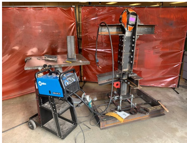
Figure 3: The sculpture during the construction process.
