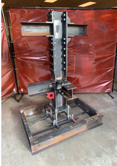
Figure 4: Steel frame sculpture ready to pour the concrete.
