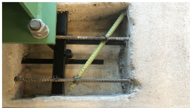
Figure 7: Lecture Slides and the Rebars and Concrete part of the Sculpture
