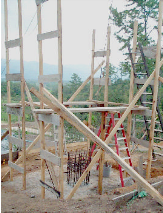
Figure 2: Scaffolding status at the end of day one (left); column rebar placement (right).
