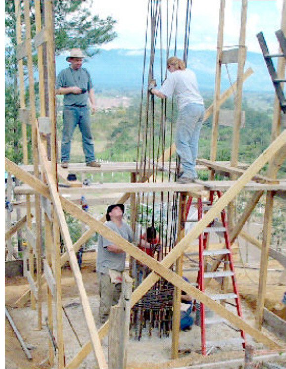
Figure 2: Scaffolding status at the end of day one (left); column rebar placement (right).
