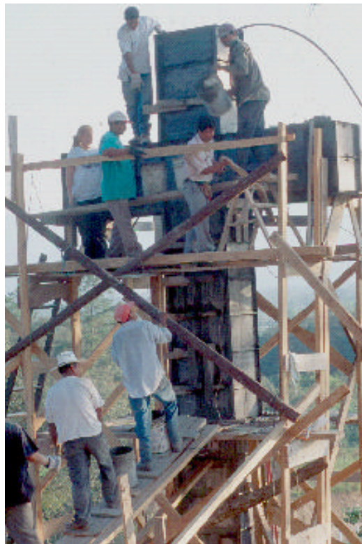
Figure 7: Placement of concrete in 5 gallon bucket increments.
