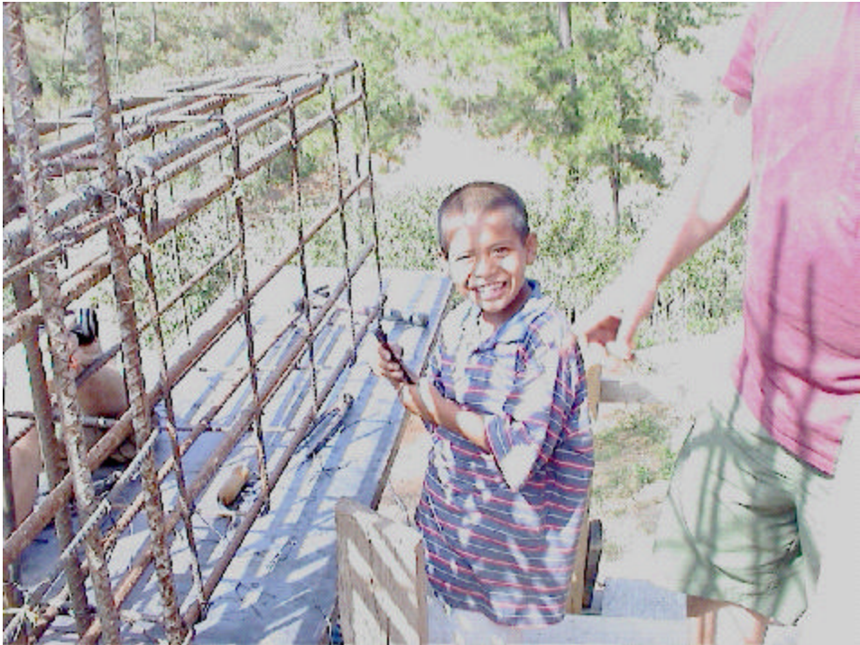
Figure 5: A “little helper” expedites the rebar placement of the cross-beam.
