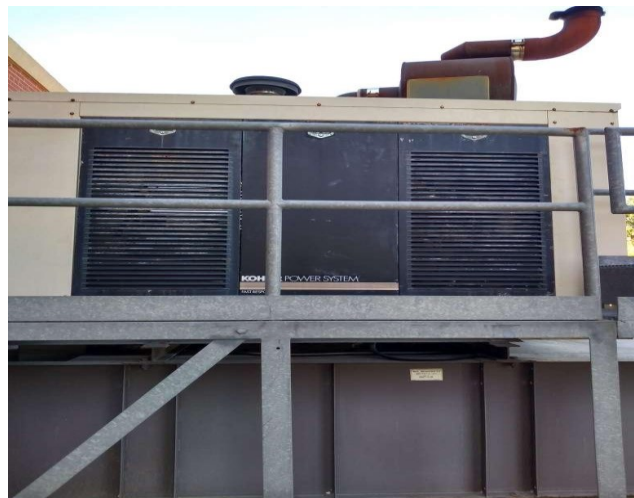
Figure 4: Emergency Generator
