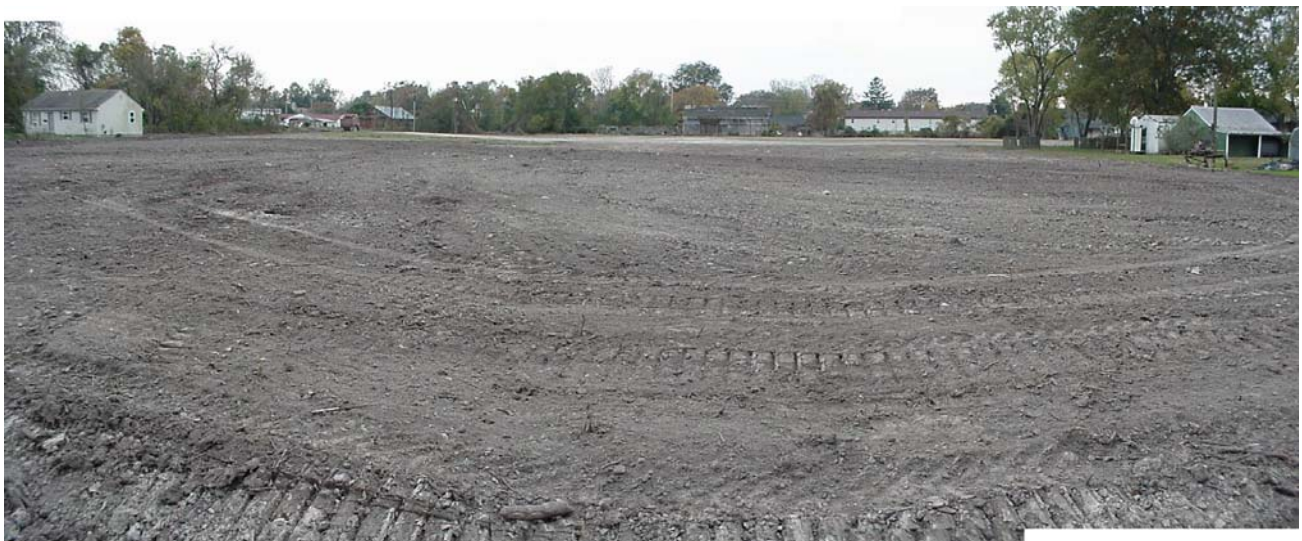
Figure 8 Completed Demolition and Site Clearance Phases
