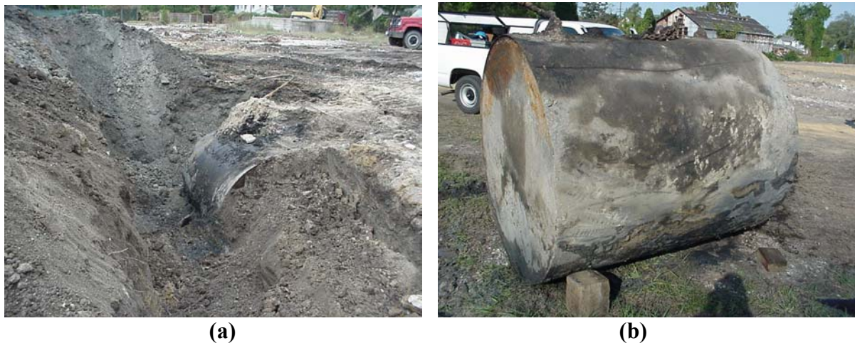
Figure 9 The Buried Heating Oil Tank
