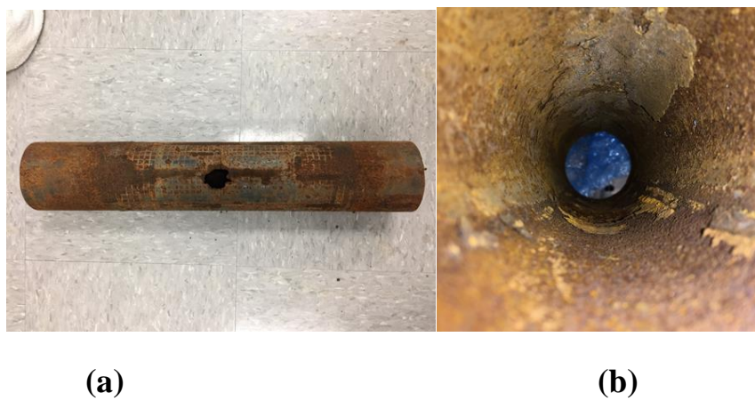
Fig. 6: External part of a API-5L Grade B low carbon steel pipe (a) and corresponding internal image (b).
