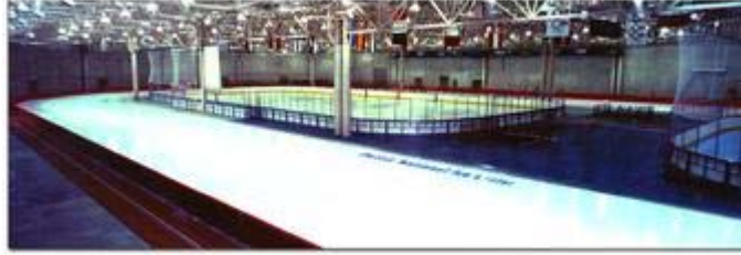
Figure 1. The Pettit National Ice Center in Milwaukee, Wisconsin.
