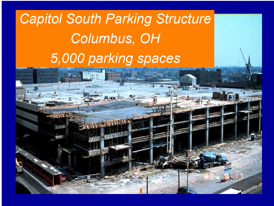
Figure 2: A silica fume concrete structure Photo courtesy of the Silica Fume Association
