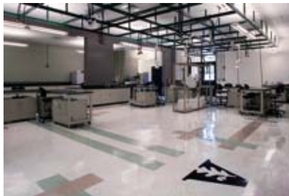
Figure 2. Photograph of the renovated space taken from approximately the same spot as that in Figure 1.
