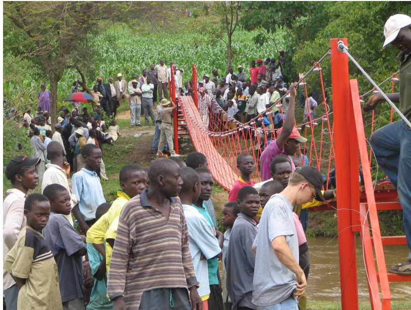
Figure 1—Building a 135 foot long pedestrian bridge over the Nzoia River in Kenya
