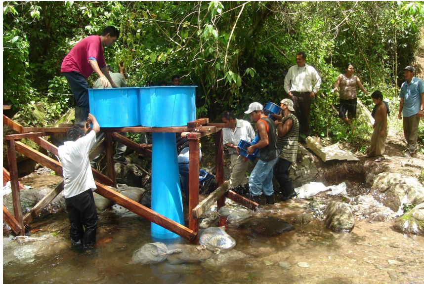
Figure 5—Installing a micro-hydroelectric generation system in Honduras
