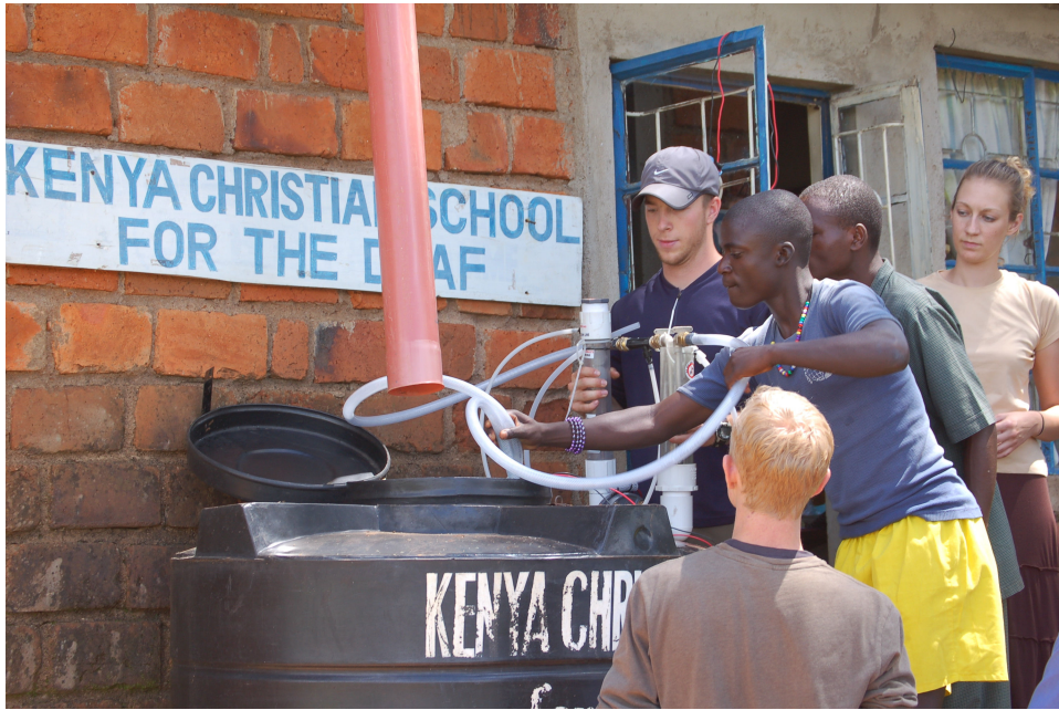
Figure 2—Installing the water purification system
